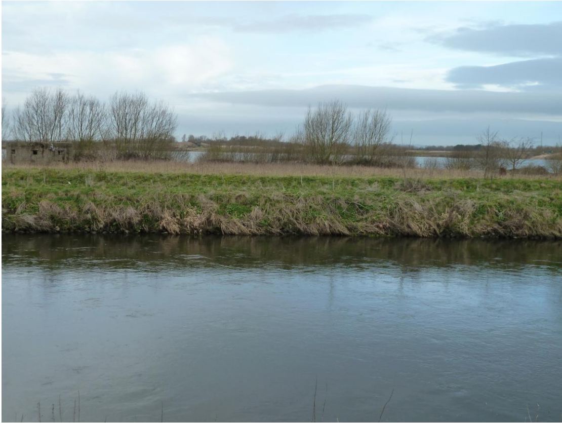
Figure 1-10: Raised bank level through deposited dredged material
