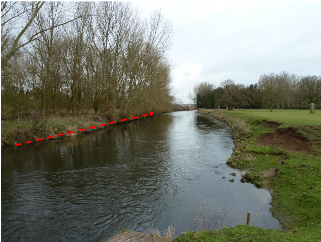
Figure 3-3: Left bank at Cherry Holme, opportunity to lower level and reconnect floodplain
