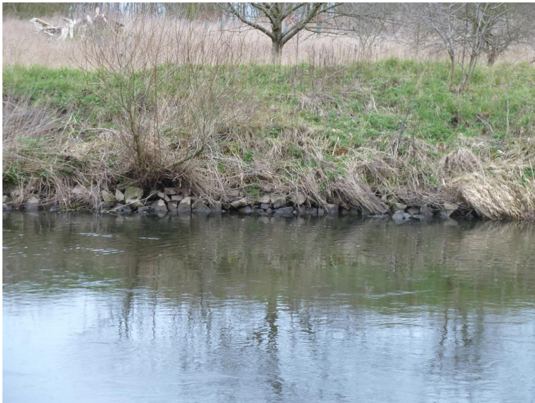
Figure 1-3: Stone pitching providing bank protection
