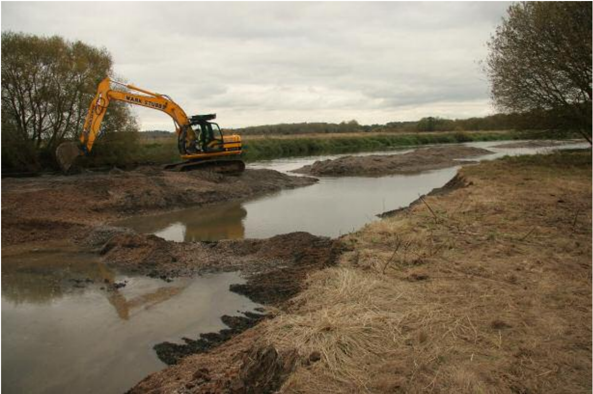
Day 30. Using gravels to form low gravels bars and islands.
