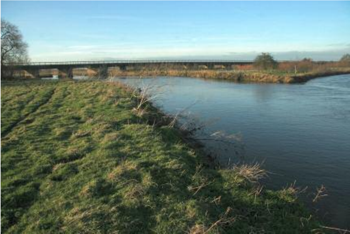
View of Tame-Trent confluence at Croxall Lakes in February 2008. Prior to the scheme being implemented.
