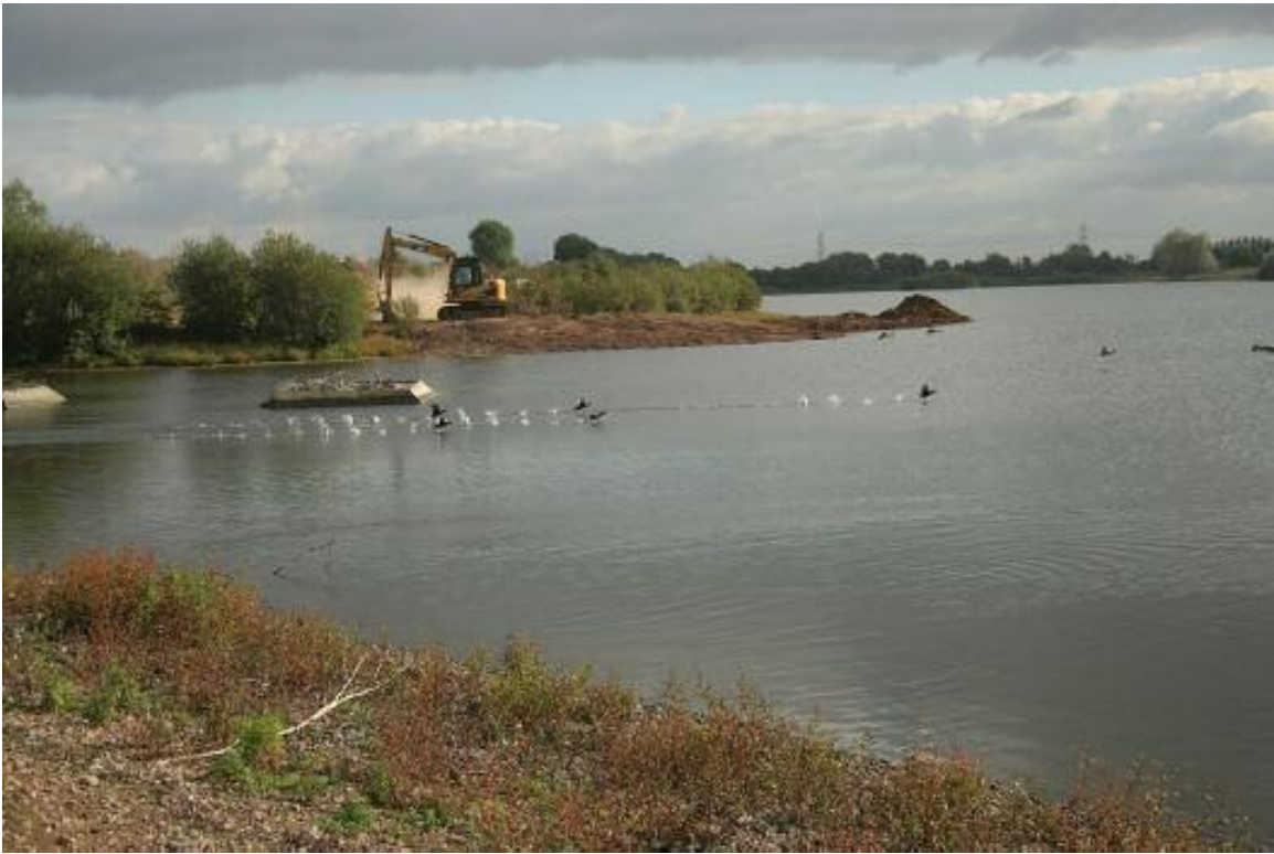
Day 6. View of deposition area in Lake 1 to create new shallows for the establishment of a reedbed.
