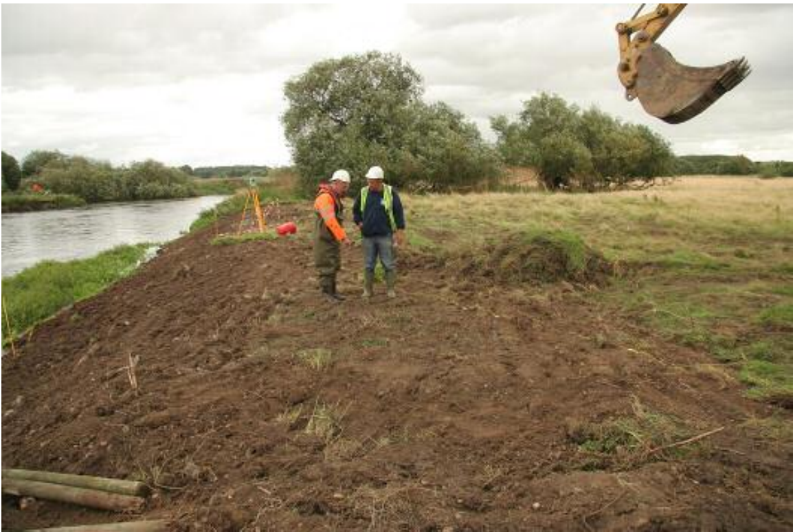
View near confluence on Day 1 of Capital Works.
