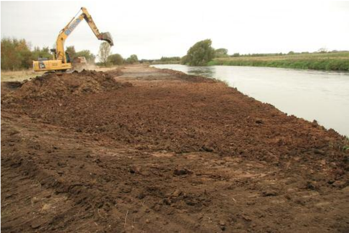
Day 20. Stripping back to expose gravel seam.
