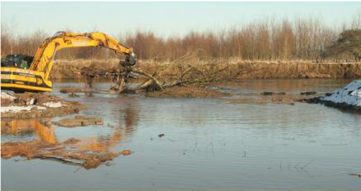
...Placing the living willow tree Large Woody Debris (LWD) with the root plate facing upstream.
