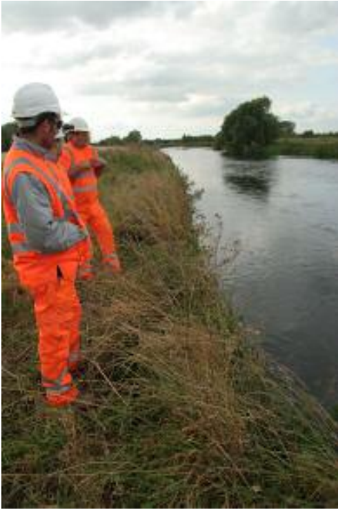
Steep, dry, engineered river banks on the R.Trent at Croxall before re-profiling.
