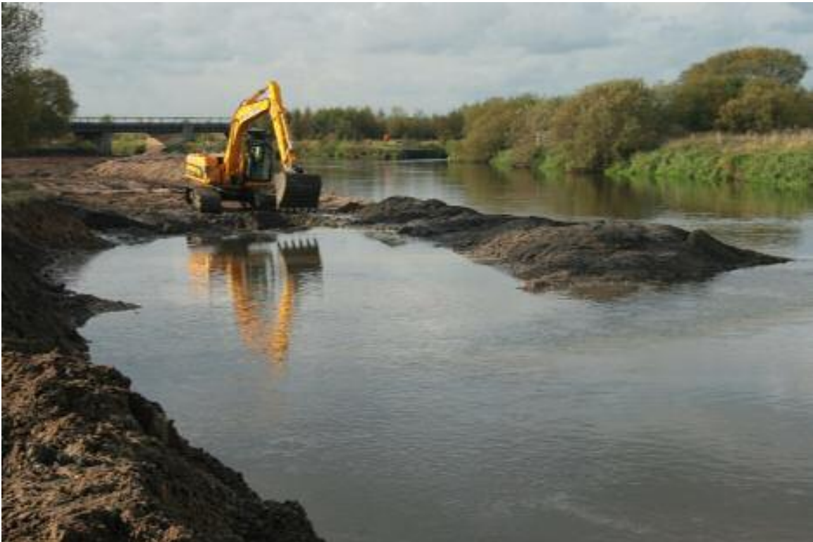
Day 30. Demonstrating technique for creation of gravels bars and islands.
