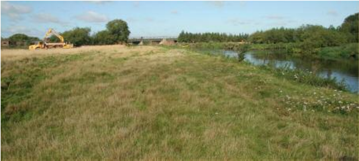
Day 3. View before river widening.
