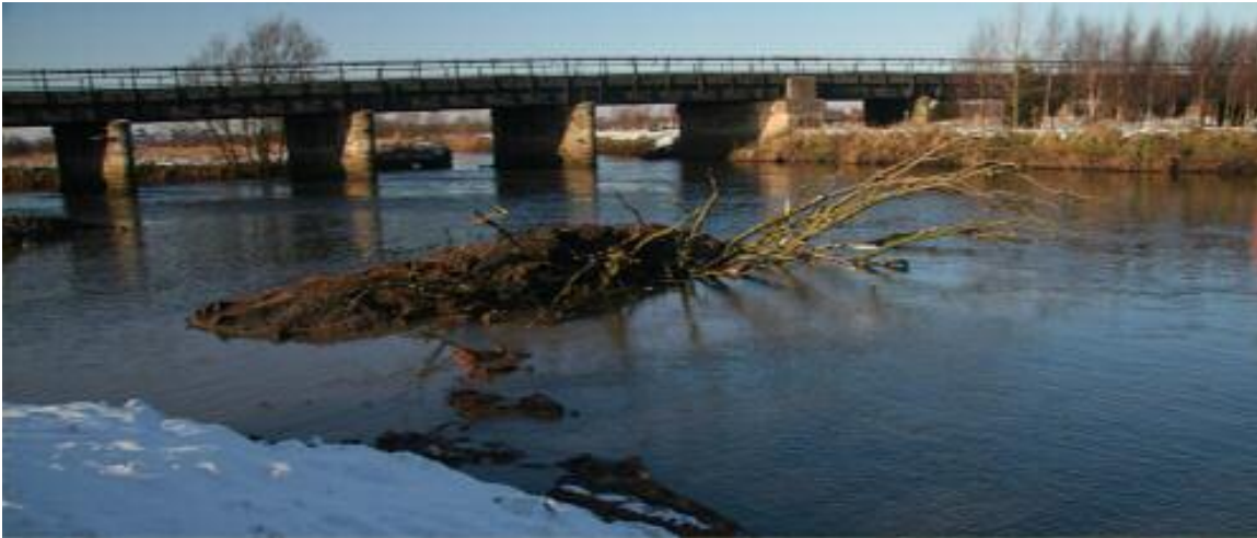
View of the newly created river island. If successful the willow will send adventitious roots into the river substrate and grow steadily. The new island will also affect deposition patterns in the river channel to generate new complexity. It should provide additional opportunities and habitats for a wide range of species including otter, depressed river mussel, white-clawed crayfish, eel, Atlantic salmon and a variety of bird species.
