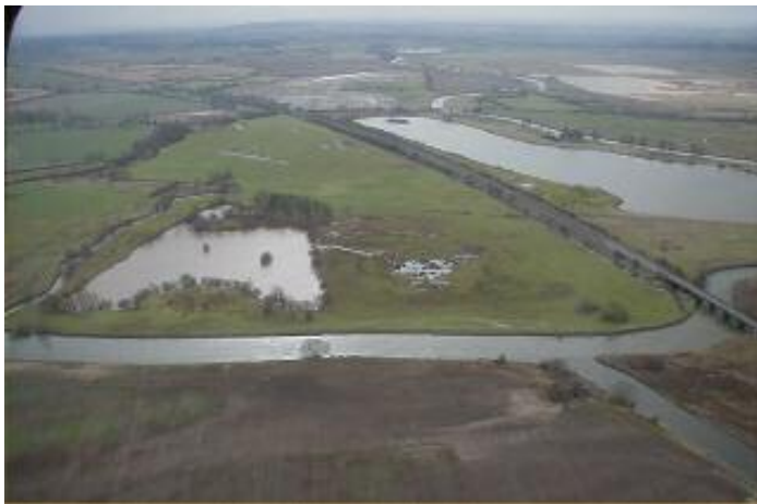
Aerial photo of Croxall Lakes in March 2003 prior to scheme being delivered. Notice the engineered character of the three main rivers. Photo © and courtesy of The Environment Agency.
