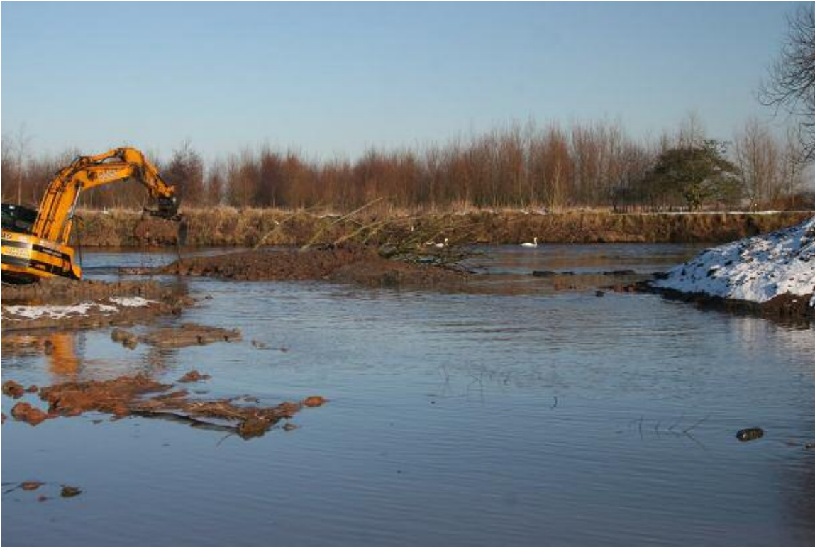
...gravel on top of the LWD and the clay.
