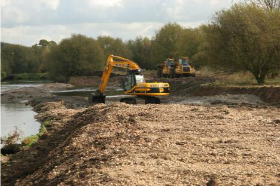
Day 30. Using retained gravels to create bars, lagoons, spits and islands.
