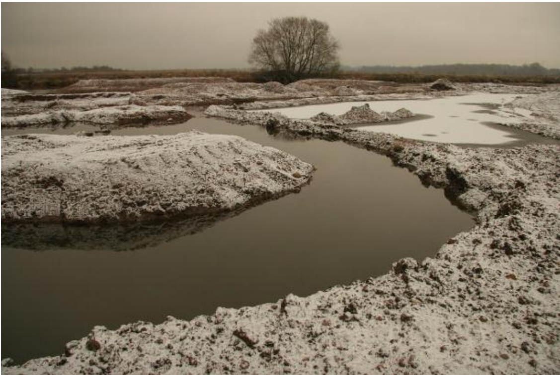
Day 86. Fine detail of the widened channel showing lagoons, perched pools, backwaters, spits, gravel bars and islands.
