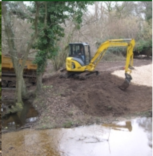
A new channel was excavated and river re-profiling carried out.
