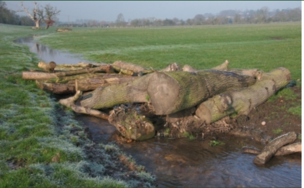
One of the constructed log jams along the newly diverted brook.
