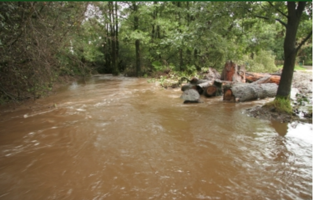
September 2009. It works! Just two weeks after the ELJ had been completed, a late summer storm resulted in spate conditions. The position of the ELJ re-activated an old channel. It is estimated that, at the peak, a third of the River Churnet's flow was diverted into this former channel.
