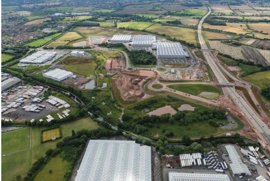
Photo: i54 site with sustainable drainage area providing amphibian habitat in the foreground
