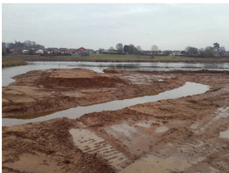
Photo: New islands being formed in Cresswell Flash, Jeff Sim
