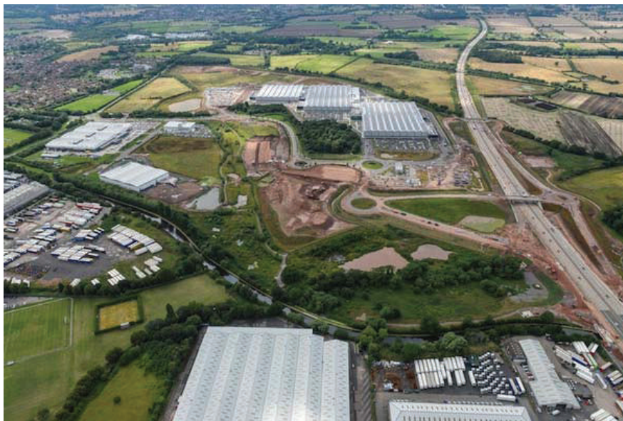
Photo: i54 site with sustainable drainage area providing amphibian habitat in the foreground
