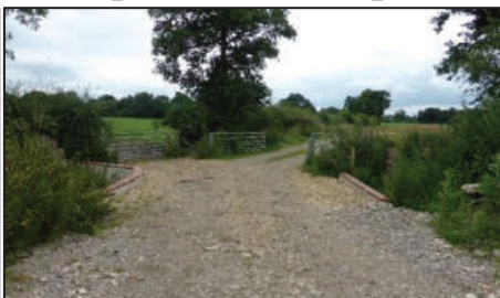
After (August 2016): Improved trackway
