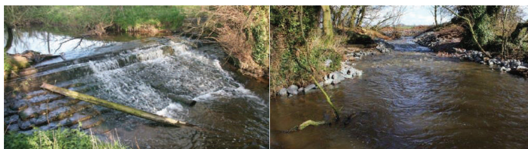
Gayton Mill Weir before, and after removal, April 2014, © Nick Mott
