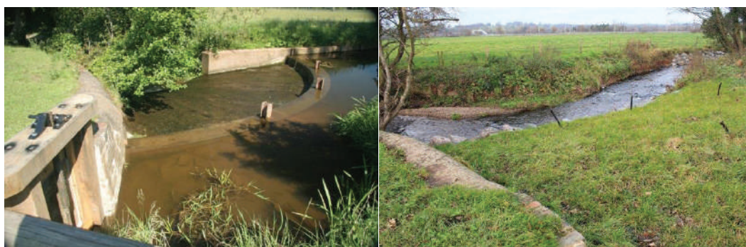
Photos: Weston Weir before (left; June 2010) and after (right; November 2013) removal, © Nick Mott
