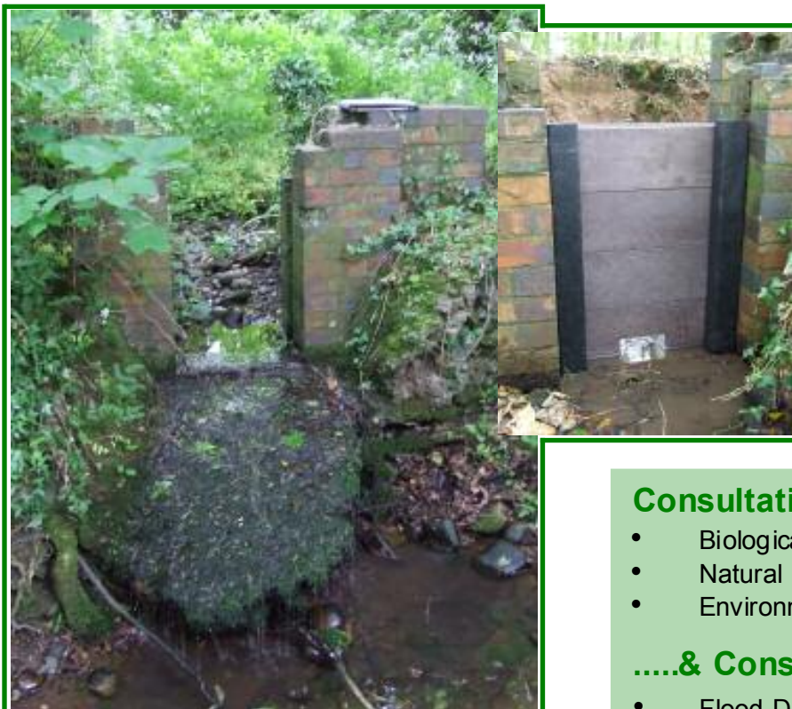
Relict brick pillars, and new water control structure
