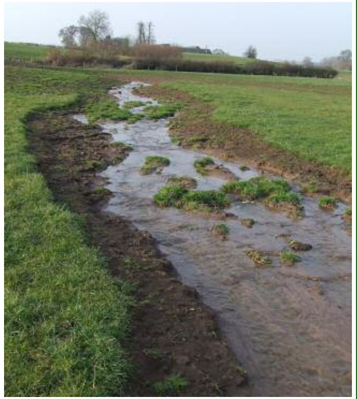
New channel, immediately after works and flowing with water
